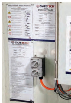
Operational & procedural signage on internal wall
