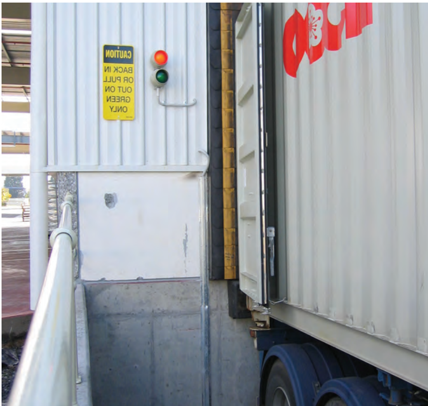
Safetech Dock Seals in use providing an effective environmental seal
