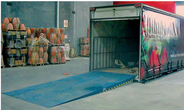
Recessed Finger Dock with typical (model 714) Dock Leveller in action, bridging the height variance between trucks and loading dock floors
