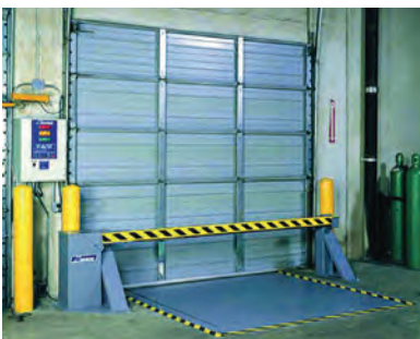
Effective traffic barriers – prevents pedestrian and equipment roll-off and door damage
