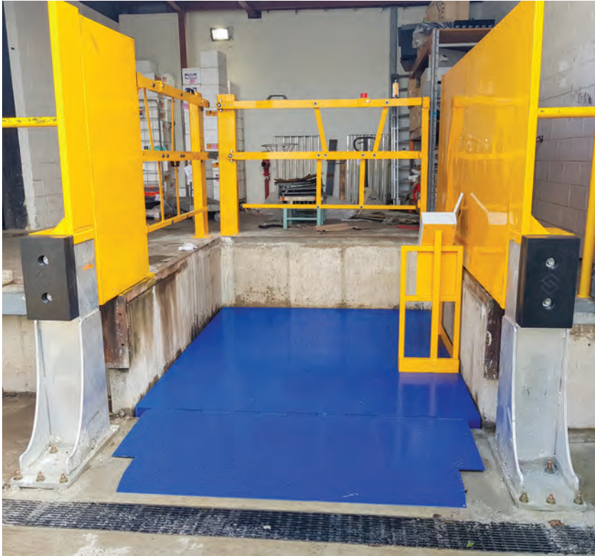
Safetech Dock Scissors Hoists allow for safe loading and unloading for trucks of all heights
